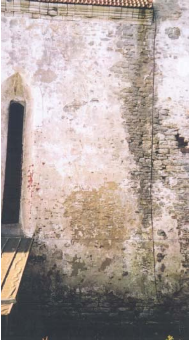
The research area on the northern façade
